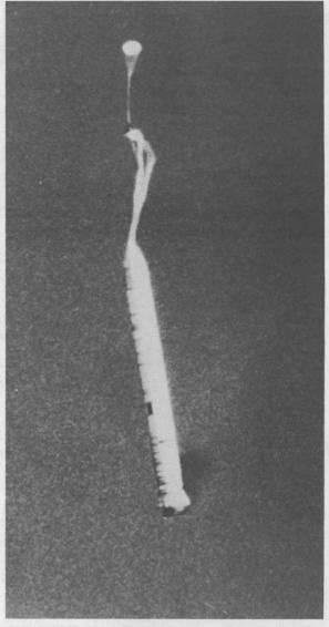
TUMBLING TO EARTH at 500 feet per second, a NASA solid-fuel rocket booster (SRB) begins its chute sequence from 16,000 feet above sea level. The pilot chute (top) and nose cap are seen here ejecting from the SRB's frustrum. The photo was taken by Navy aircraft after a shuttle launch in 1983.
